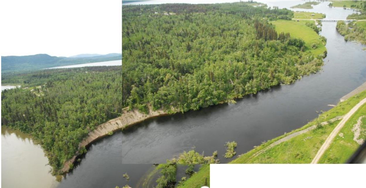
Photo 6.1 Photo of the confluence of the Nechako and Nautley rivers taken on June 26, 2007, showing backwatered conditions on the Nautley River. The discharge at WSC Nechako River below Cheslatta Falls (08JA017) and Nautley River near Fort Fraser (WSC 08JB003) was approximately 548 m 3 /s and 169 m 3 /s, respectively. The Nechako River is seen on the left, the Nautley River is on the right, and the photo is facing upstream. Source: M. Miles and Associates (2007b).
